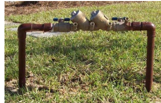
Example of a backflow prevention
