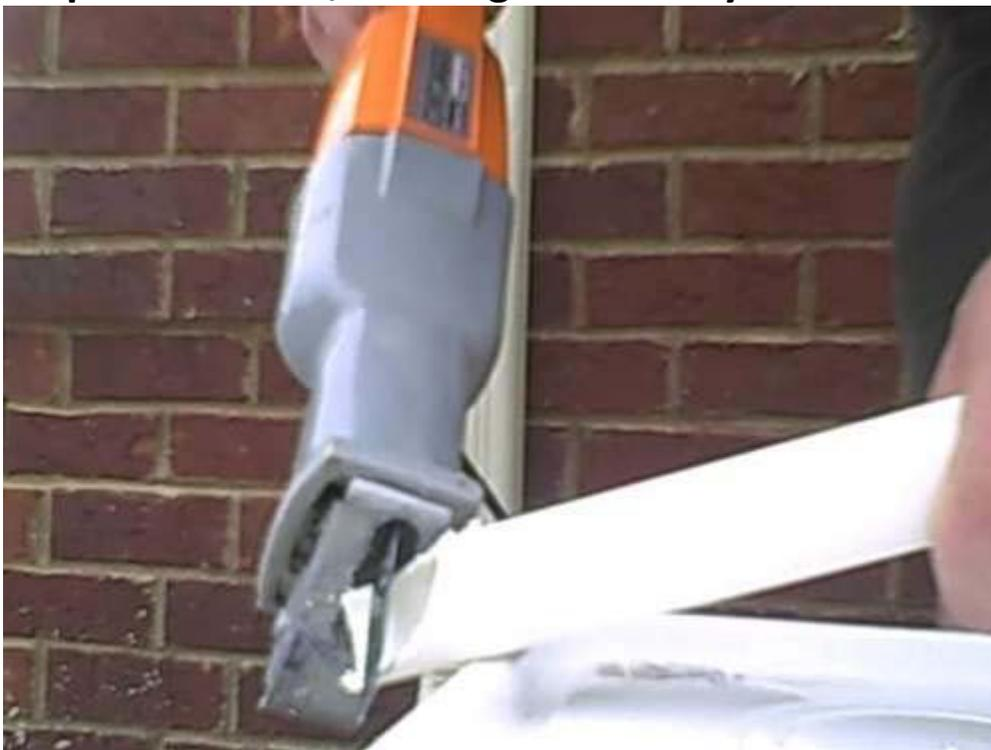
Cut your 1" pvc so that it is long enough to reach from the bottom of your box and stick out a few inches. Notch/Wedge the end if you like to make sure it won't sit flat on the bottom and get clogged.
